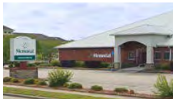
Gulfport North 14245 Dedeaux Road
